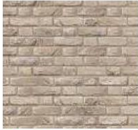
1 Buff brick in Flemish Bond
