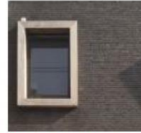
7 Timber window surround
