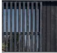
5 Vertical dark coloured timber screen & cladding
